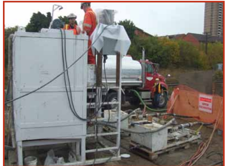
Utility Services, Cellular Grouting, Toronto, Ontario Light weight cellular grout is used to backfill casings after delicate conduits and high voltage cables are installed beneath railroad tracks, airport runways or roadways.
